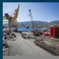
QUAY UPGRADE deepening, widening
